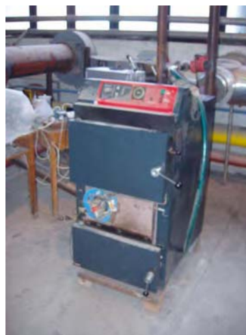
Obr. 2 Kotel na tuhá biopaliva V 25 Fig. 2 Boiler for solid biofuels V 25
