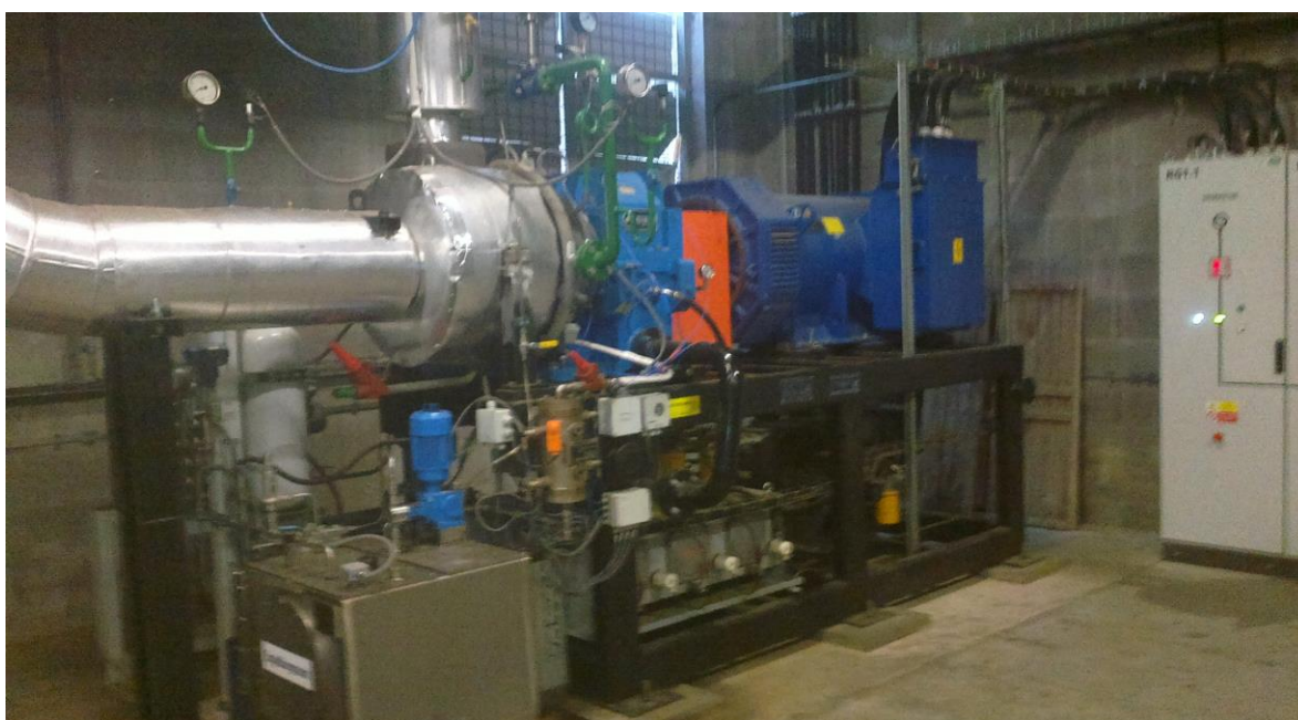
Obr.2: Turbina ORC 600
