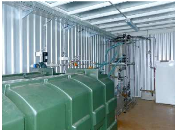
Fig. 16: View of the part of operational set of cooling and cleaning of syngas line VÚZT, v.v.i. Prague - PolyComp, a.s. Poděbrady with containers for operational liquids and condensation waste and washing column of raw syngas
