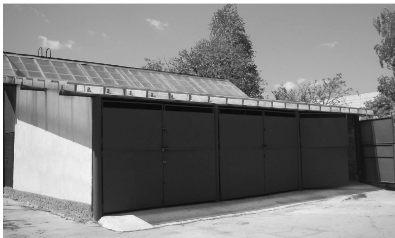
Fig. 2. Overall view of the experimental biomass dryer
