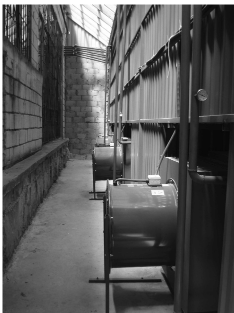
Fig. 3. Mixing chamber with reversible fans
